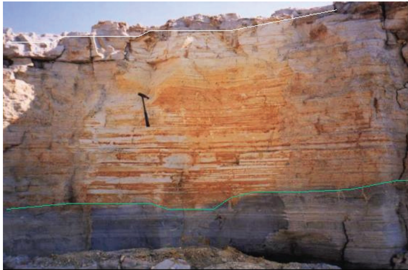
Figure 2.3: Typical oxidation zone profile (~4 m high) in ERGO 5L29 dam
