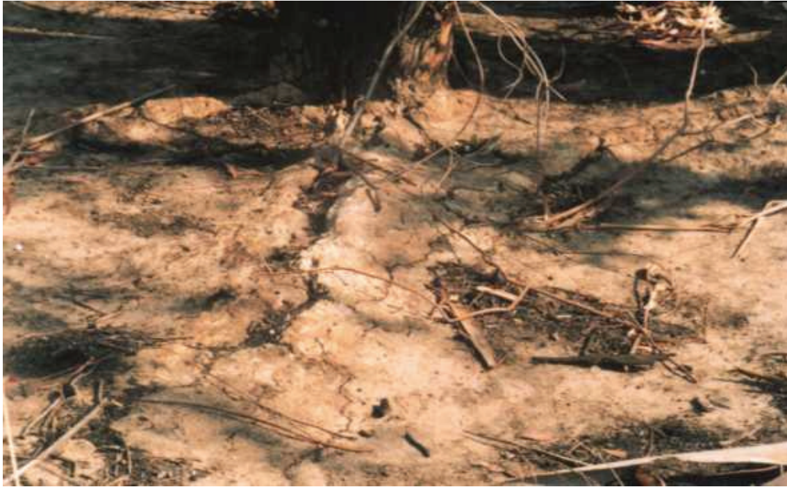
Figure 3.25b: Root-induced fractures in CMR-3L1 tailings dam
